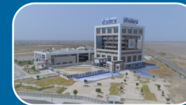
DHOLERA ABCD BUILDING
